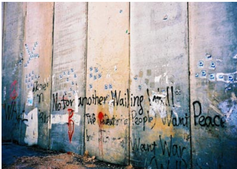
Israel's "separation barrier."
