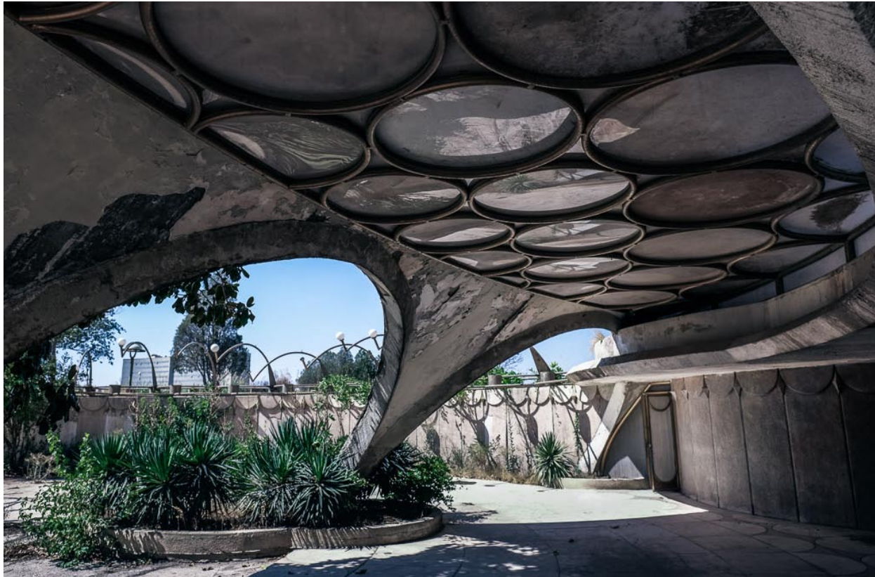
INTEGRATED: The palace featured outdoor plants in a courtyard that was integrated with the living area.
